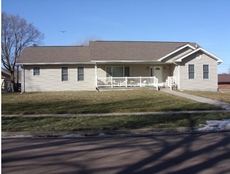
The church parsonage was built in 2003. It has a full basement, 5 bedrooms, and 3 full baths.
